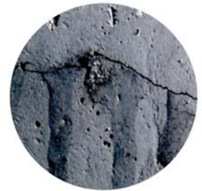
裂缝渗漏
